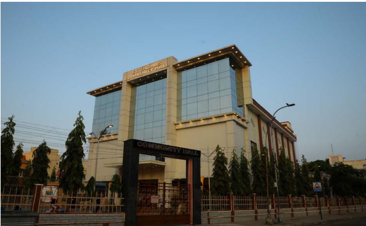
« St Thomas Community Hall » après rénovation. St Thomas Community Hall completed and reopened, Feb,2021
